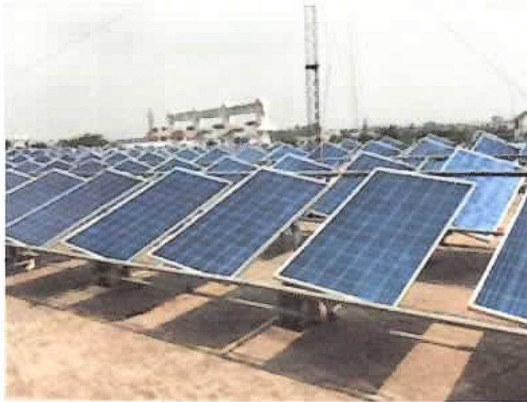
Solar Panel Installation
